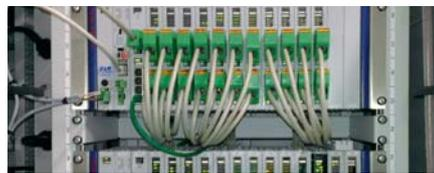
machines. Previously a net-line FW-50 station in a 19" rack was chosen with IEC 60870-5-104 connection. In addition to the relatively large I/O capacity with metered value processing and switch actuation with checkback via DSO modules, two Modbus remote connections for cogeneration plant control and a further PLC were realised.
